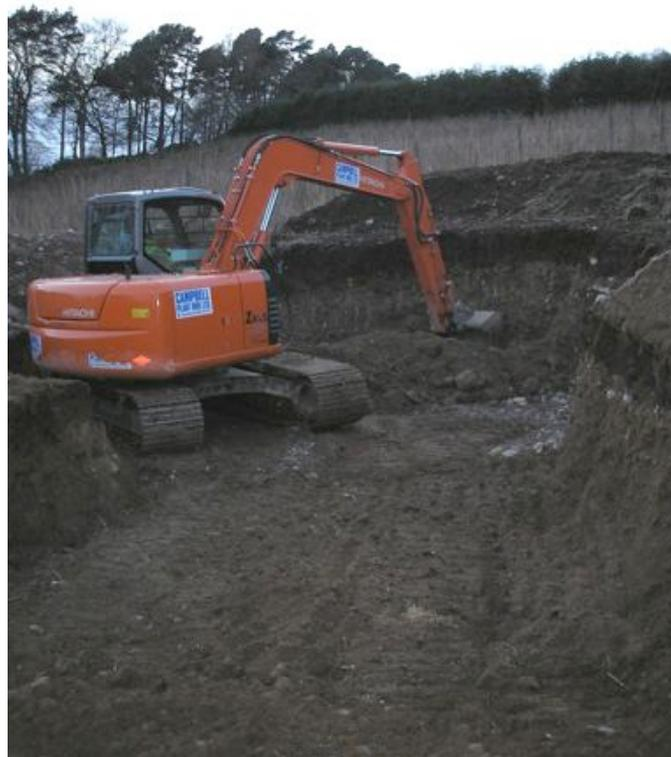
Excavation work, with a final maximum depth of eight feet the site seems well drained, although the subsoil was very hard.
