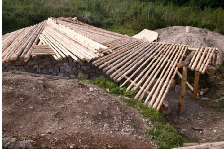
The completed roof showing the sky light, vertical supports and additional spacers close to the ring beam. The beam was thus supported in three places plus the reciprocal joining at the centre. It was roughly estimated... very roughly estimated that with the overhang beyond the wall the uprights were close to a point of weight balance on the roof.
