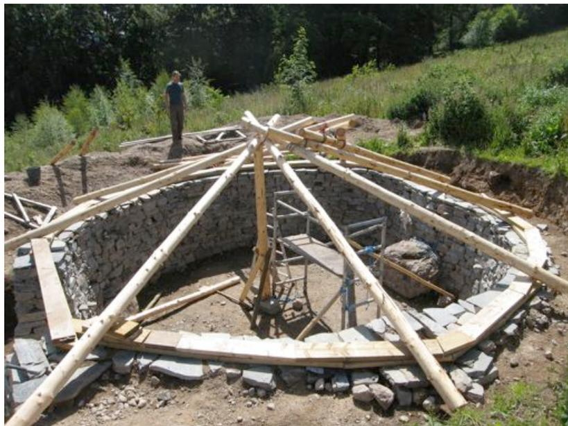
All additional roofing poles were then laid on top of one of the main poles and attached top and bottom. We were keen to have at least 1M overlap on the wall, partly to ensure water is shed well away from the wall but also to provide a counter balance for the weight of the soil covering over the main space.
