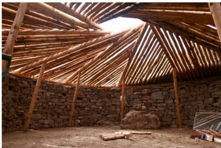
With the roofing poles secured, they were covered with a thick layer of rank heather, the woodier the better. This provided good support for an insulating layer of straw. Butyl rubber was then laid over the straw, topped with carpet to protect the rubber from the final topping of grass sods to the tune of 3-4 inches.
